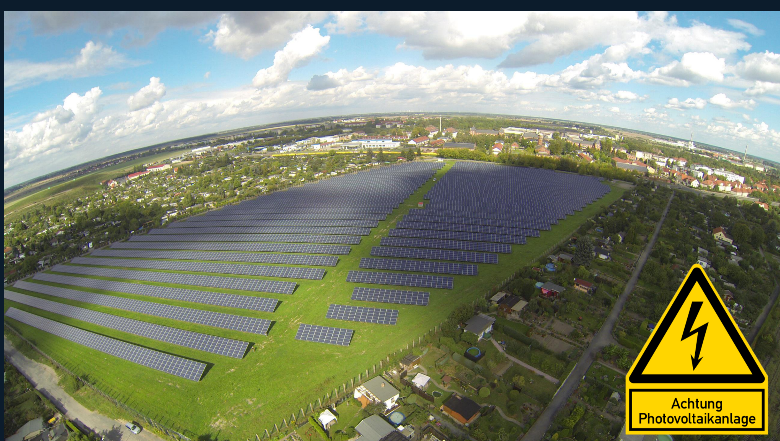
PV plant in Germany. Photo: Guillermo Oviedo
