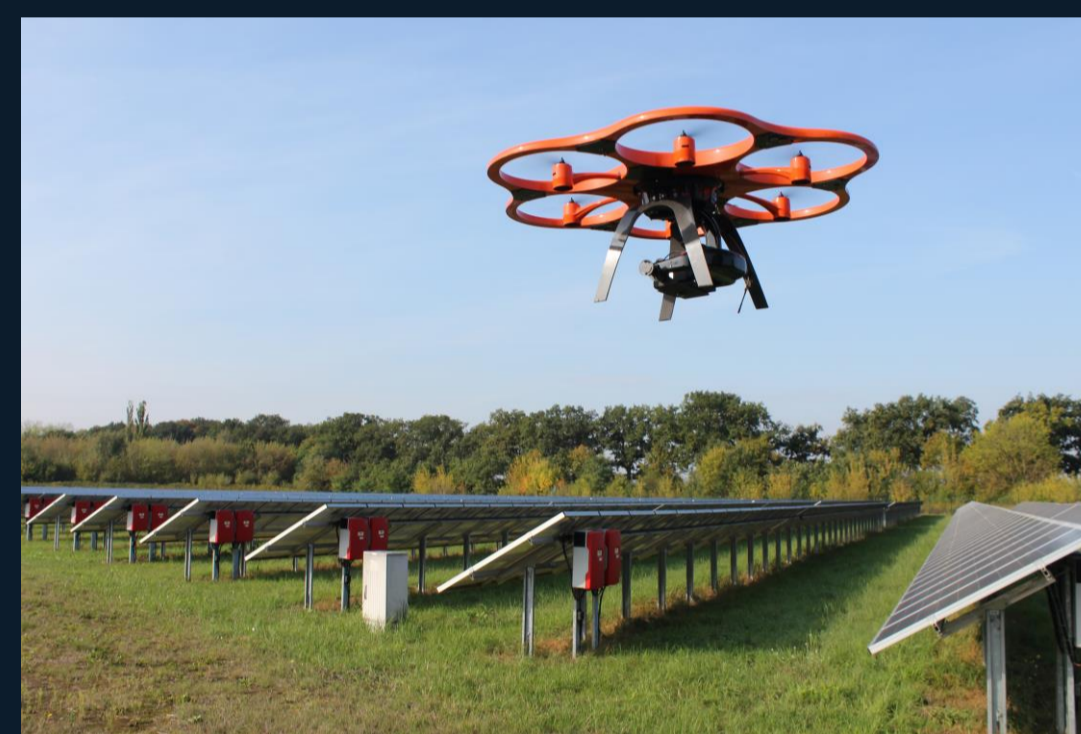
Aerial IR inspection. Photo: Guillermo Oviedo
